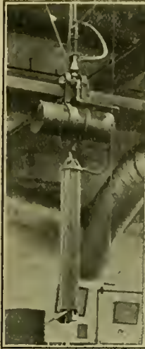
FIG. 17.—AIR HOIST IN WHEEL SHOP.
